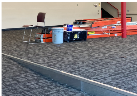
3. Raised flooring, a wheel-chair accessible ramp and carpeting were installed over electric and networking cables
